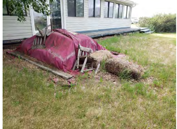
Photo 6: View of the covered septic tank on the west side of the residence (June 23, 2021).
