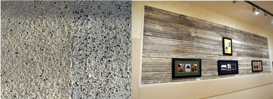
Left: close-up of stucco (hall bay left, church bay right of seam); Right: exposed wooden siding of former exterior north wall of church, now interior south wall of hall.
