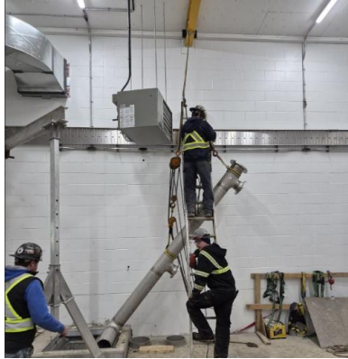
March 30 th : Site Conditions
