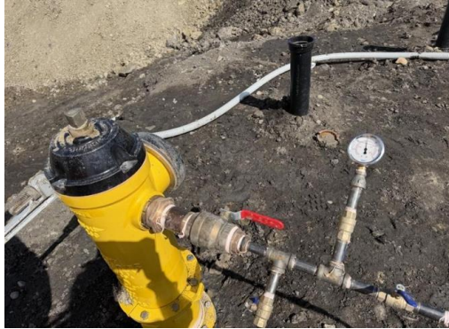
April 13 th : Pressure test
