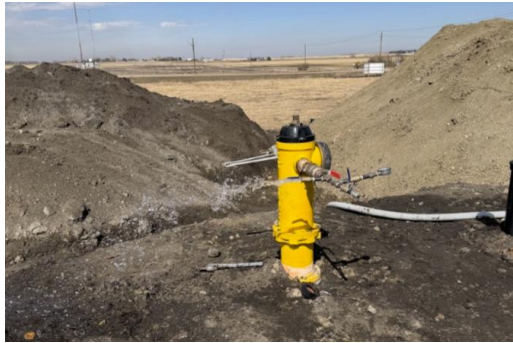
April 13 th : Pressure test
