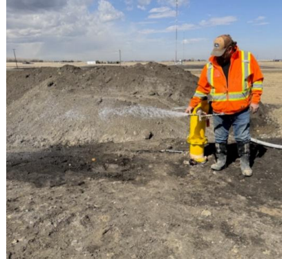
April 13 th : Pressure test
